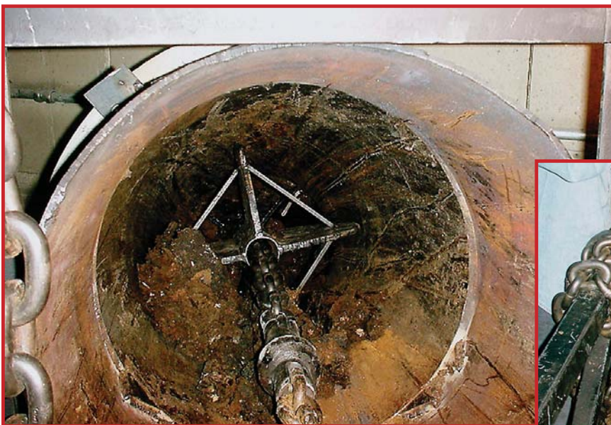
Innovations from Pipe Genie cleaned the 20-inch waste pipe at Brigham and Women's Hospital after four other contractors failed with more conventional methods.
