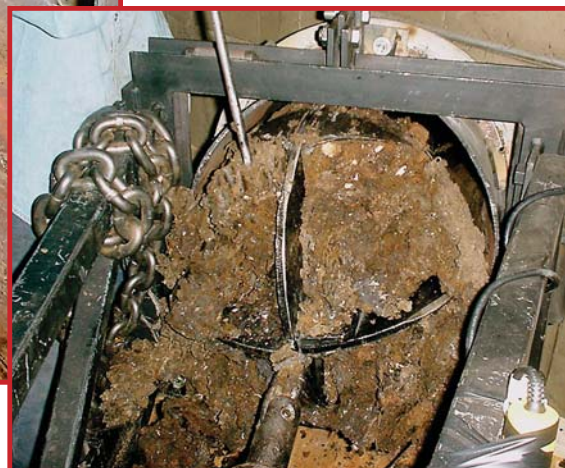
Innovations from Pipe Genie cleaned the 20-inch waste pipe at Brigham and Women's Hospital after four other contractors failed with more conventional methods.
